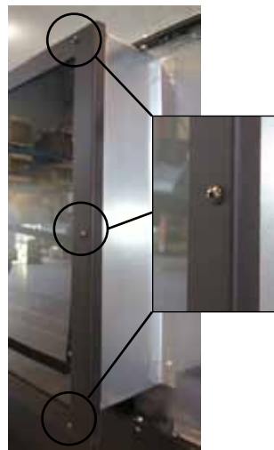
Figure 16. Step 3 (Removal of Door Frame)
